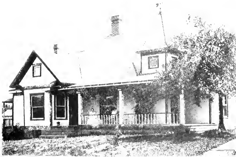
RESIDENCE OF A. W. PFEIFER, North Sixth Street.
